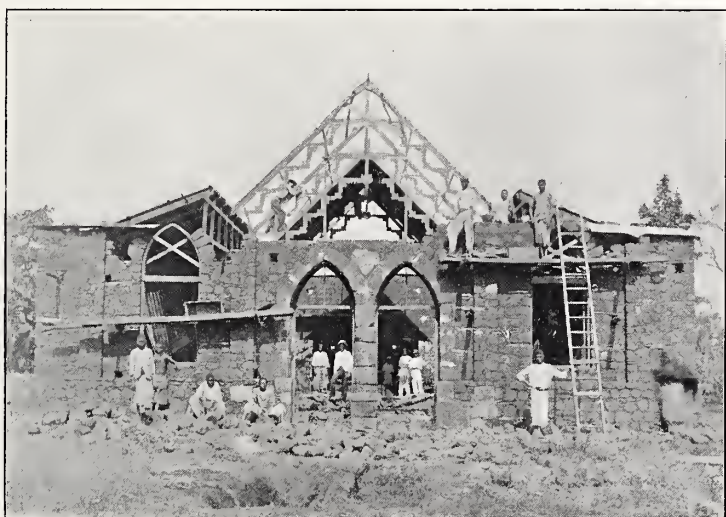
NEW MISSION CHAPEL IN BUILDING, SAN SALVADOR
